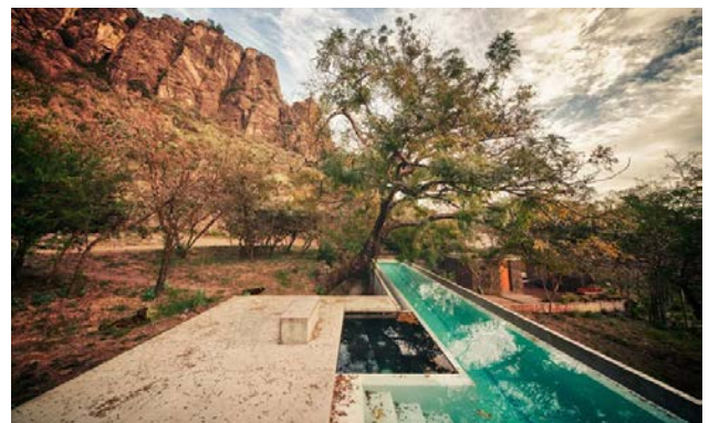
The house also features a narrow, elevated swimming pool. Water is collected on site in three large containers (the pool, a maintenance reservoir and a potable water tank) to ensure there is no waste and to allow year-round irrigation (Image credit: Press)
